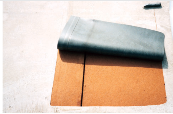
Plaza Towers Atlanta, Georgia
