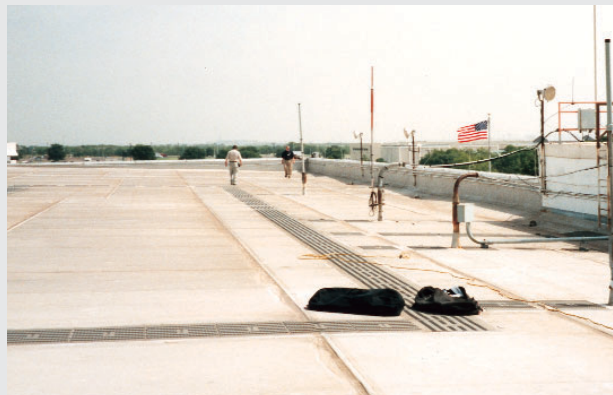
Federal Aviation Administration Building Eules, Texas
